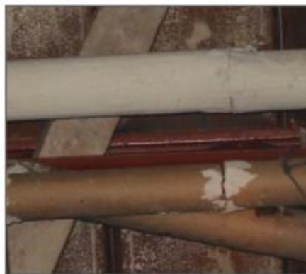
Parging cement on sweatwrap and Aircell
