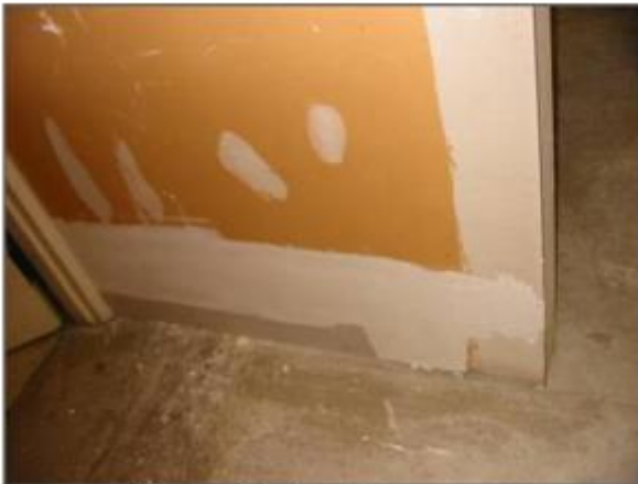
Compound on drywall
