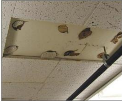
Glued on (laminated) ceiling tiles
