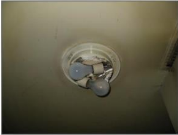
Paper heat shield on incandescent fixture
