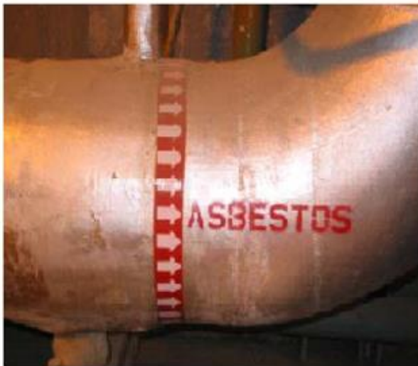
Asbestos Marking
