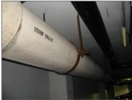
Transite Drain Pipe
