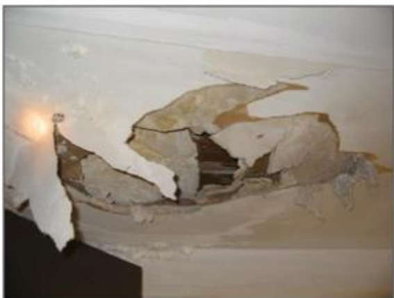
Plaster on wood lath
