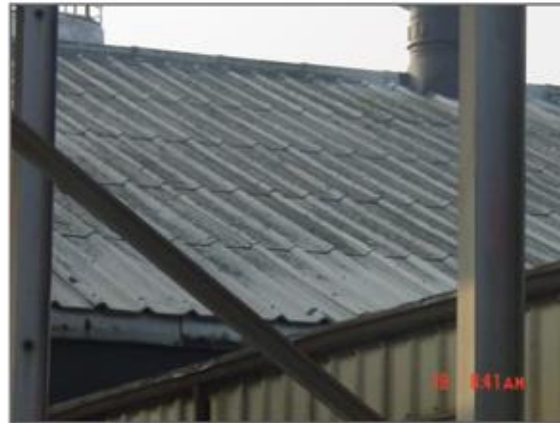
Corrugated Transite Siding/Roofing
