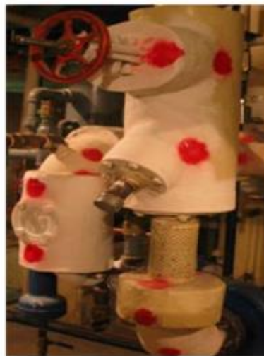
Asbestos Markings
