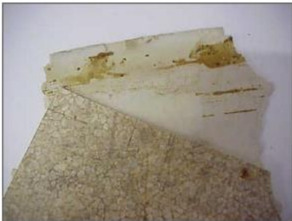
Vinyl sheet flooring with paper underneath
