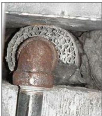
Aircell insulation (corrugated paper)
