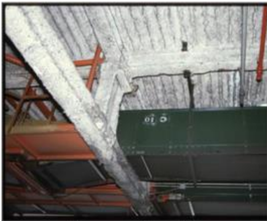
Fibrous sprayed fireproofing
