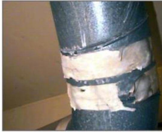
Paper on seams of duct
