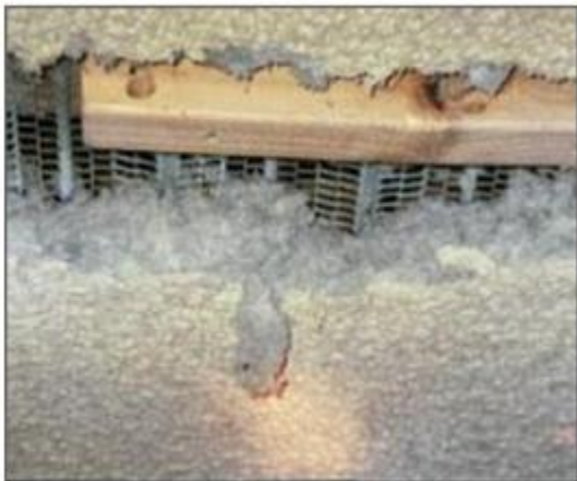
Sprayed limpet texture ceiling on lath
