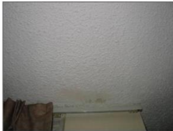
Texture coat ceiling
