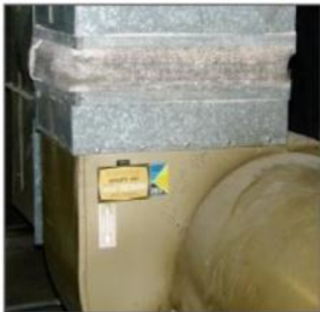
Textile Vibration Damper/Duct Connector
