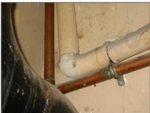
Parging cement on pipe fitting
