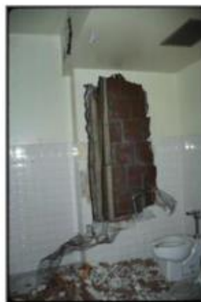
Plaster on speed tile
