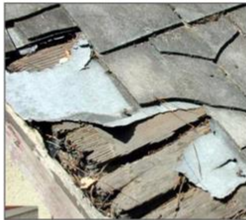
Building paper under roof tiles
